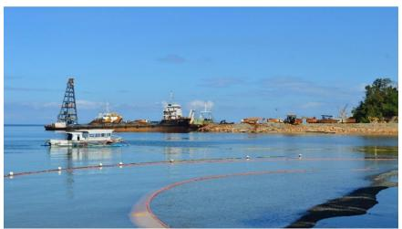
4 Silt curtains and floating rafts installed underneath the barge ramp surround the Agata Causeway to catch possible debris, and thus mitigating siltation in Tubay's waters.
