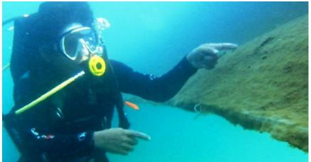
**3** AMVI Environment Manager Jesalyn Guingguing shows how a cordon of silt curtains made of geotextile fabric and inter-woven abaca coco-nets effectively trap silt and debris under water.
