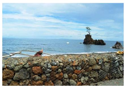
1 Several Gabion Baskets fortified with Coco-nets and or Geotextile fabric installed surround AMVI's Port and Causeway area serve as a barrier designed to trap silt and other unwanted debris from reaching the coastal waters of Tubay.
