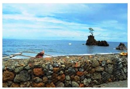
4 Several Gabion Baskets fortified with Coco-nets and or Geotextile fabric installed surround AMVI's Port and Causeway area serve as a barrier designed to trap silt and other unwanted debris from reaching the coastal waters of Tubay
