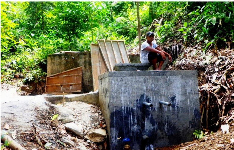
1 On-going construction and system upgrade of Barangay Tinigbasan's water system.
