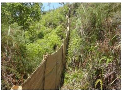
2 Silt fences made from interwoven abaca sacks are installed along slopes to keep sediments and debris from flowing down the mountain and entering the rivers.
