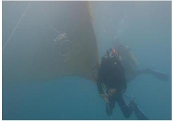
**1** A company-trained diver installs the coco net silt curtain around the causeway area to prevent silt from floating into the ocean.
