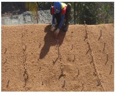
3 Company personnel install interwoven abaca sacks along slopes to serve as braces to control soil erosion.
