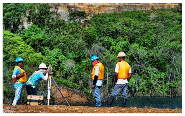
**Eyes on the ground.** TVIRD personnel survey the surrounding Canatuan tailings impoundment area to provide an update on the current elevation of the topography in order to create digital terrain models, which are also used for estimating resources and mine development plans. The company is set to bring the same successful Canatuan business model to its Agata North project in Agusan del Norte.
