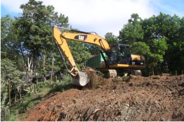
2 A backhoe strengthens the soil directly above the Agolo area.
