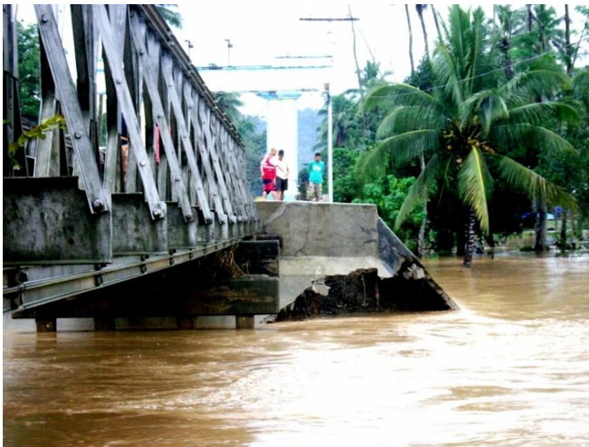
3 The northern approach of the town's Mendiola Bridge - Siocon's oldest bridge – is not spared from the destruction brought by massive rainfall.
